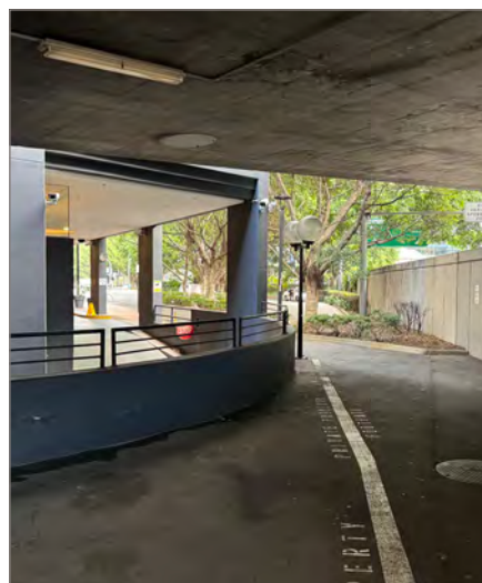
8. Under Western Distributor
