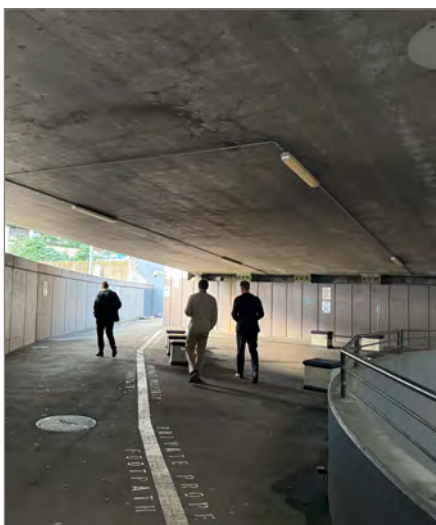
7. Under Western Distributor
